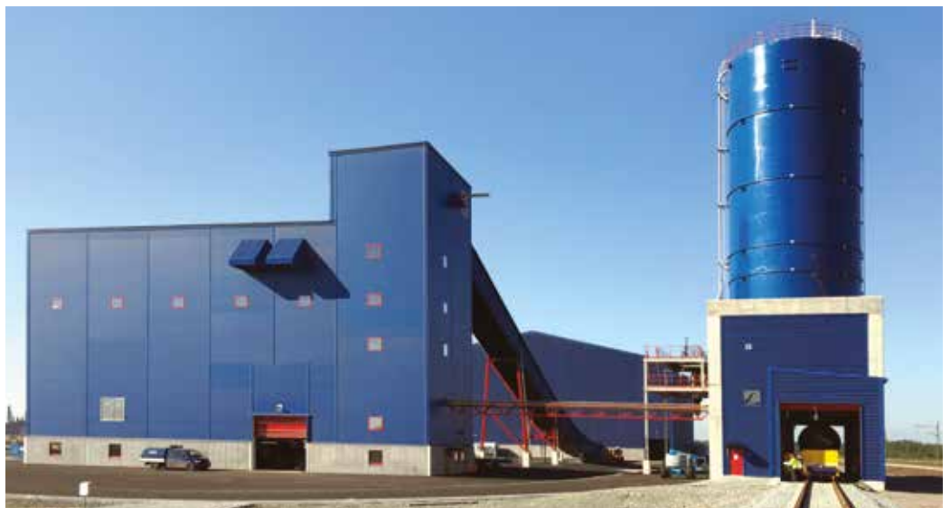
Bentonite grinding plant with dispatch silo.
