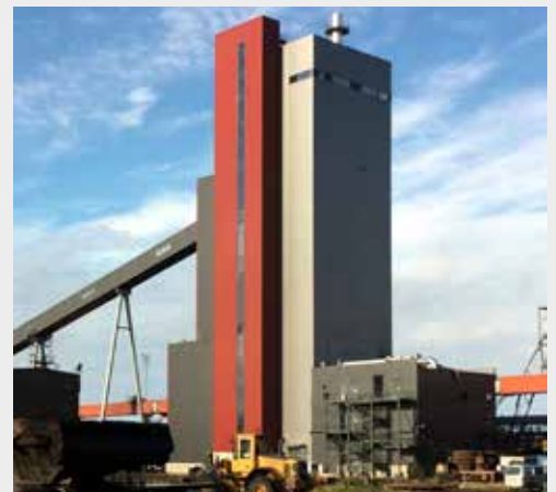
Coal grinding and injection system for 2 blast furnaces.
