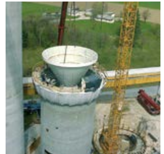
Erection of the CC silo.
