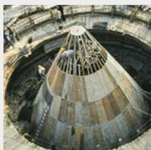
Expansion chamber under construction.
