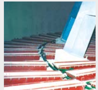
Steel mixing expansion chamber, retrofitted in old silo.
