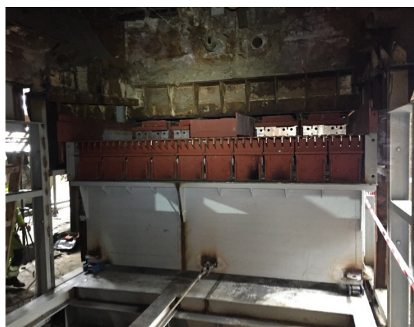
Figure 4. Pulling new modules into their final position.
